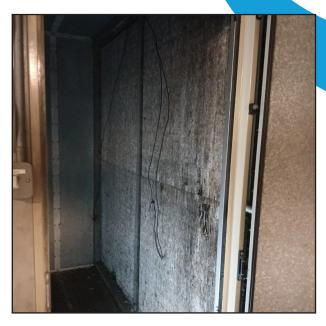
New coil, filter frames and corrosion treatment completed
